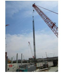
Testing of the piles was carried out from a working platform lowered onto the test pile. All gauges were read automatically using a data acquisition system. To eliminate the erection of a reference frame, pile head movement was monitored manually by digital level off the adjacent test pile.
