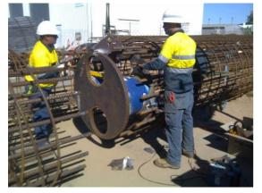
Fixing O-cell Assembly to Cage
