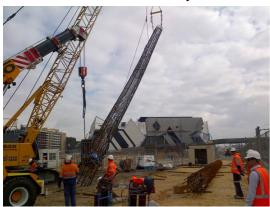
O-cell Instrumented Pile Cage Being Lifted
